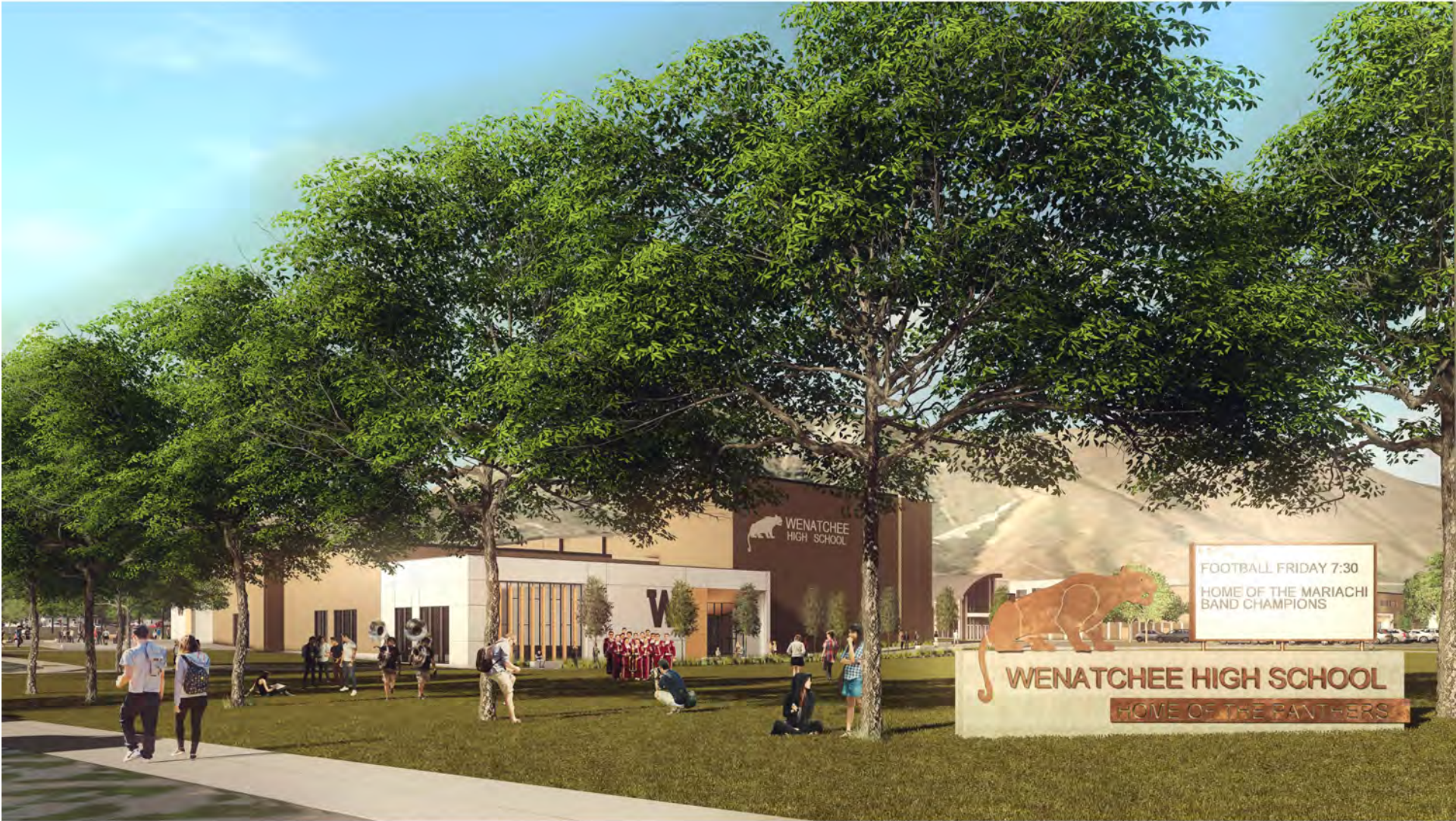
MUSIC ADDITION LOOKING SOUTHWEST
