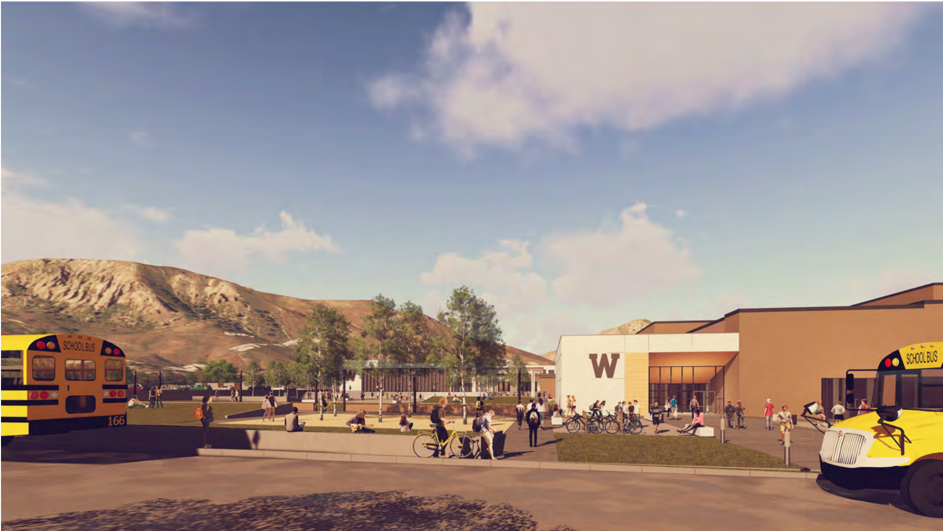
PLAZA LOOKING WEST
