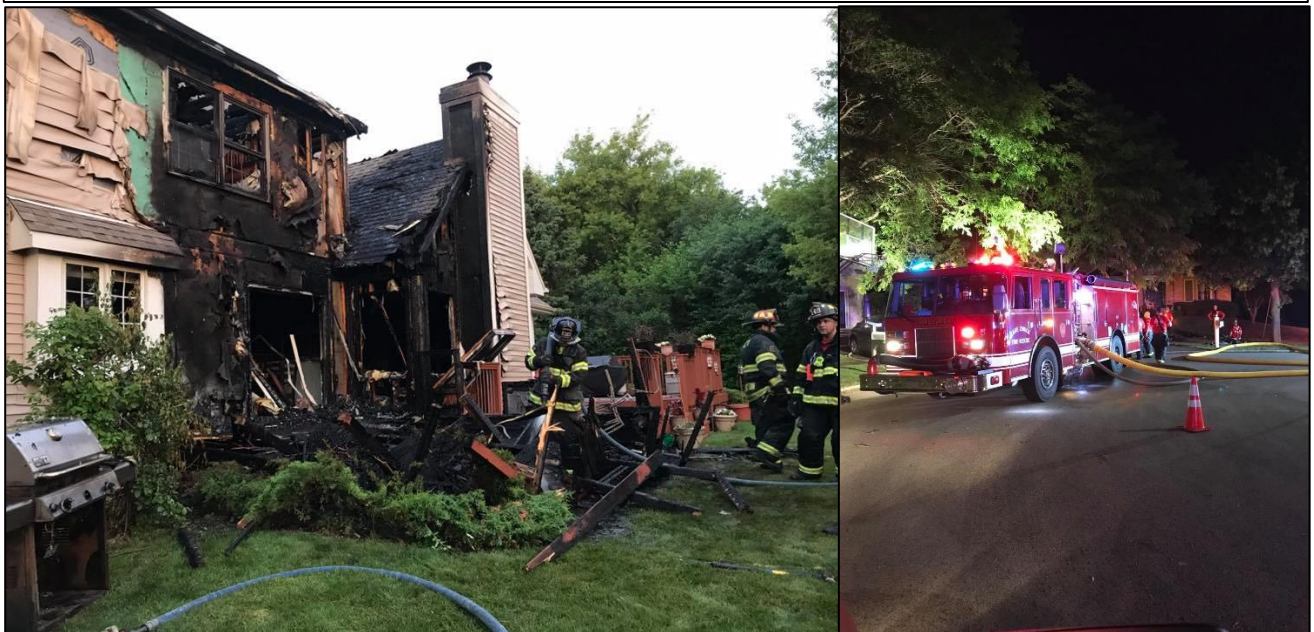
Structure Fire at 500 block of Carolian Drive (pictured above)
