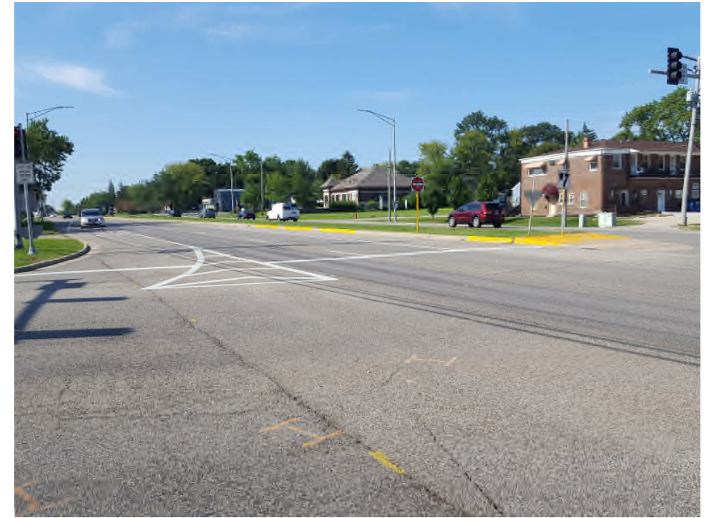
Looking south along U.S. 12 NB approach at Old Rand Rd
