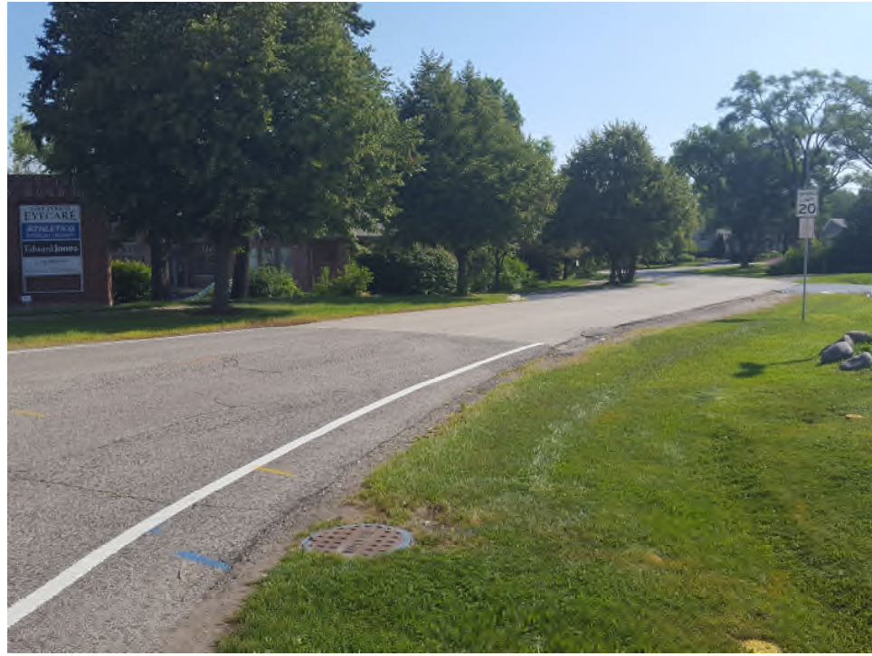
Looking east along Golfview Rd at U.S. 12
