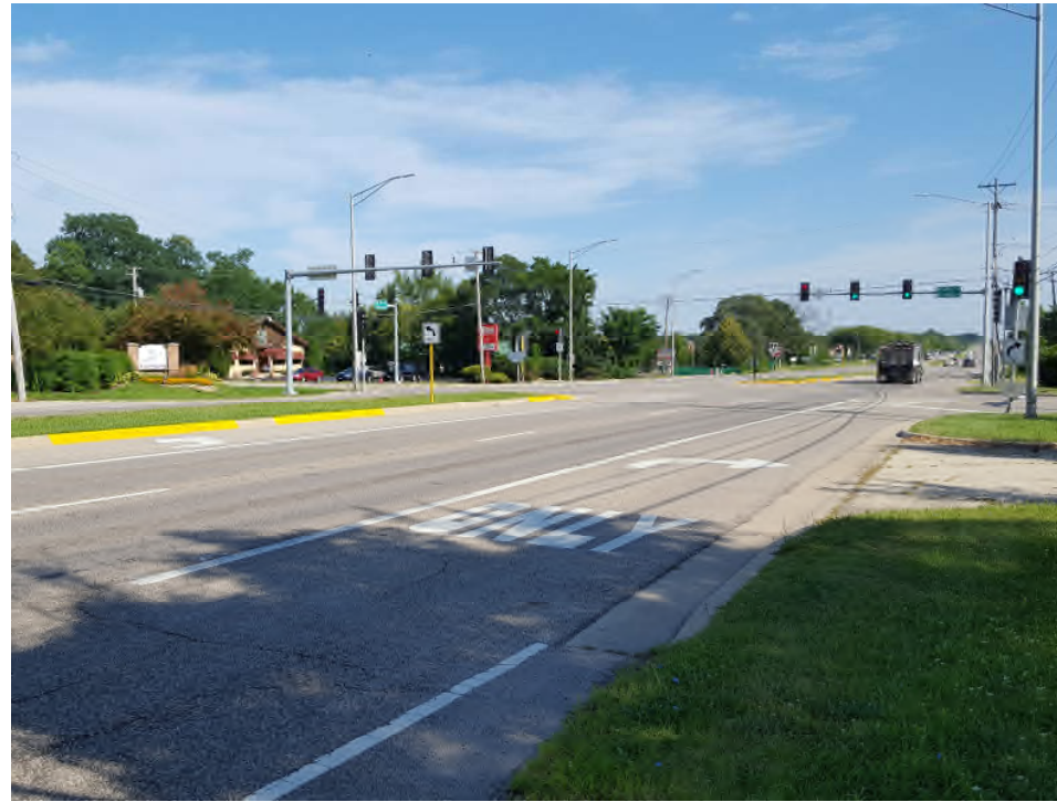
Looking north along U.S. 12 NB approach at Old Rand Rd
