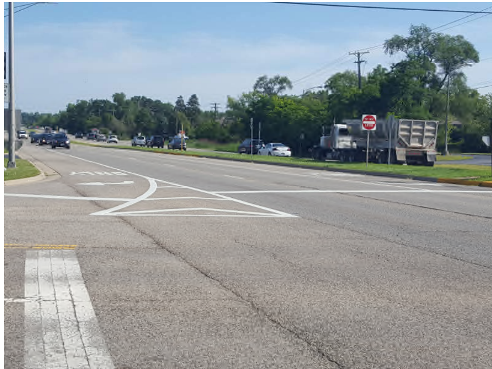
Looking north along U.S. 12 SB approach at Ravinia Terrace
