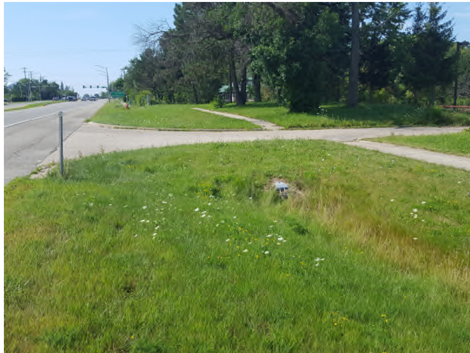
Looking south along U.S. 12 SB at Golfview Rd lot entrance
