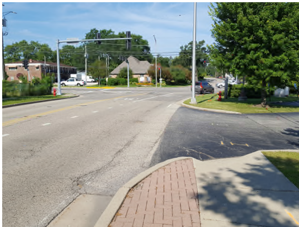
Looking west along Old Rand Rd approach at U.S. 12
