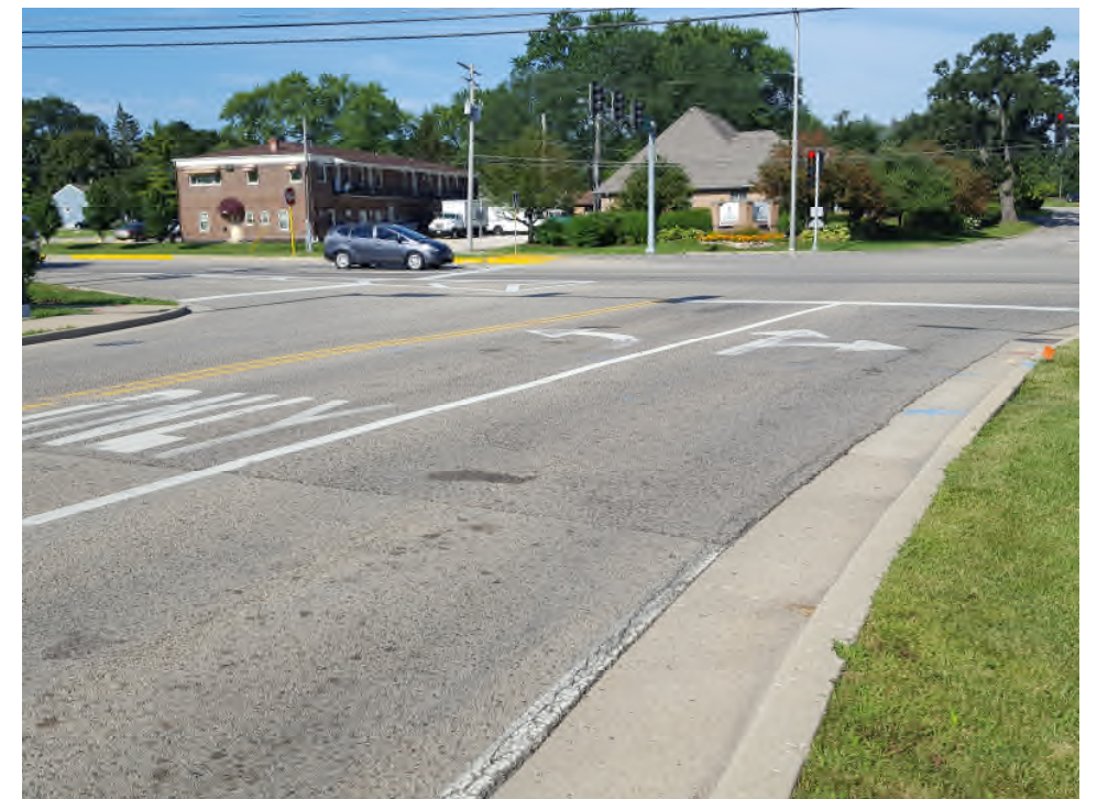
Looking west along Old Rand Rd approach at U.S. 12
