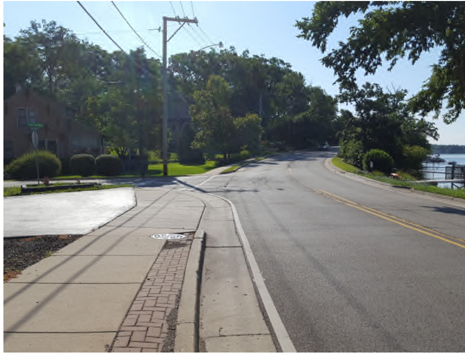
Looking east along Old Rand Rd at Pine Tree Row
