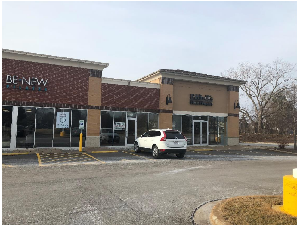
Figure 3: Facing south from Rand Road towards the vacant tenant space that the existing massage therapy business proposes to occupy.
