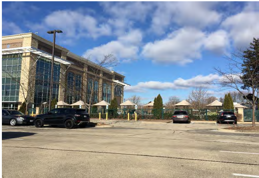
View looking north showing east elevation of main building and outdoor pool/cabana area
