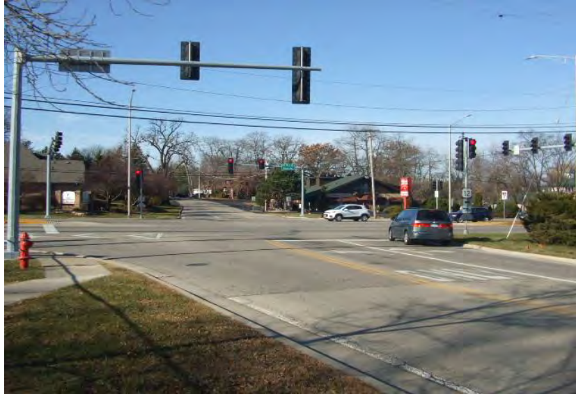
View looking west from Old Rand Road at subject's signalized intersection
