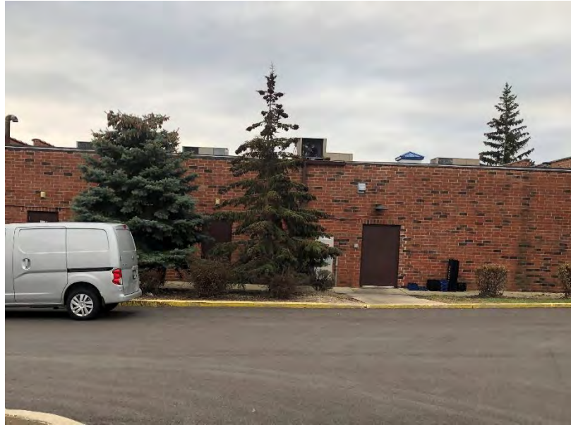
Figure 5: Looking south towards the rear of the adjacent commercial building from the Subject Property.
