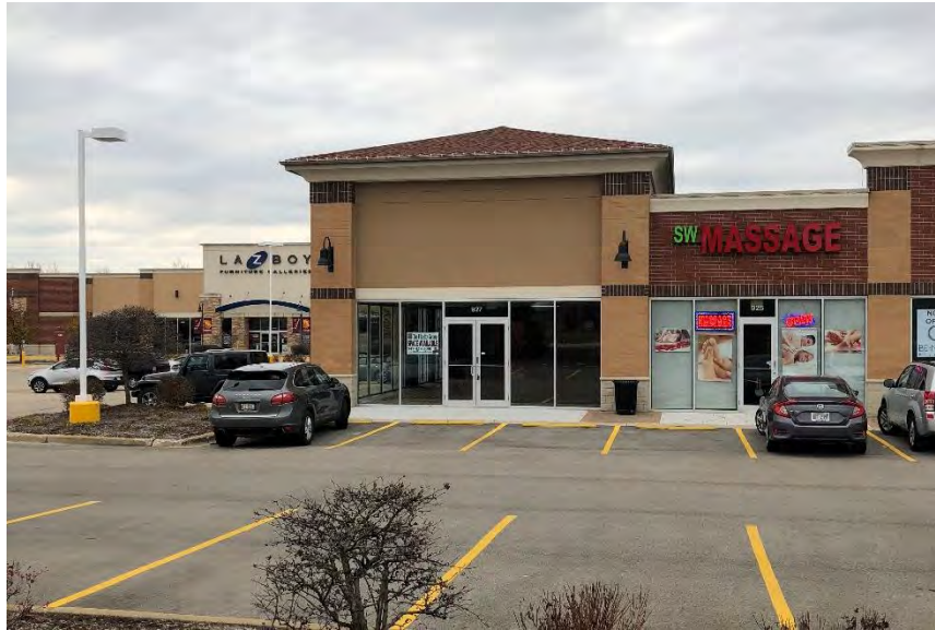
Figure 1: Facing south from Rand Road towards the Subject Property.
