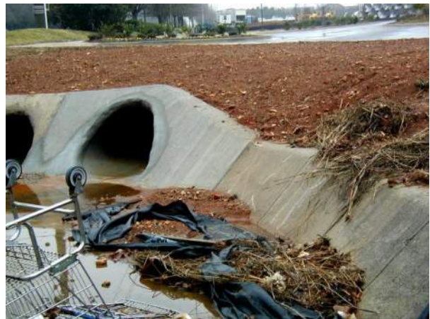
The impact of erosion from construction sites is controlled by straw bales and silt fences. Proper emplacement and maintenance of these measures is vital to keep channels clear.
