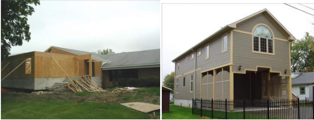
The WDO requires major improvements to existing buildings and all new building to have the lowest floor including the basement elevated to the Flood Protection Elevation (FPE), which is 2 feet above the base flood (or 100-year) elevation.
