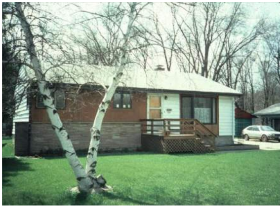
This house was elevated one foot above the base flood elevation of the Des Plaines River (prior to the adoption of the WDO).
