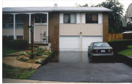
Houses with drive-down garages are susceptible to street flooding and local drainage problems
